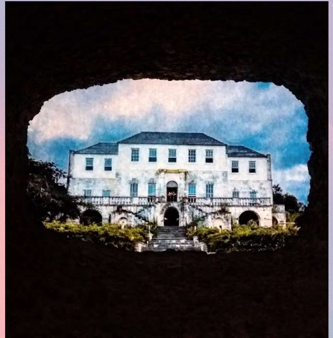
Work in progress. Rose Hall Estate
